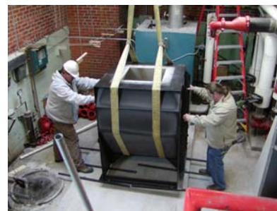
Installing the pellet burner.
