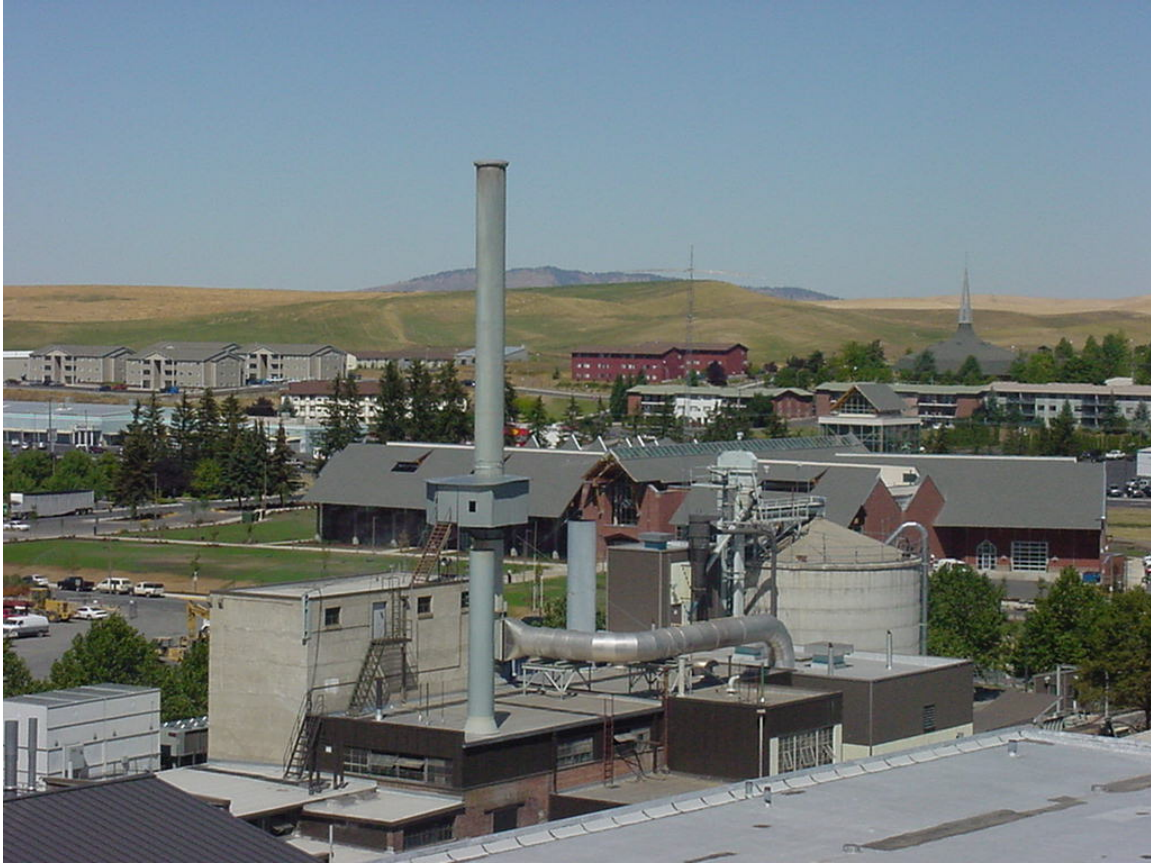
University of Idaho Boiler Plant
