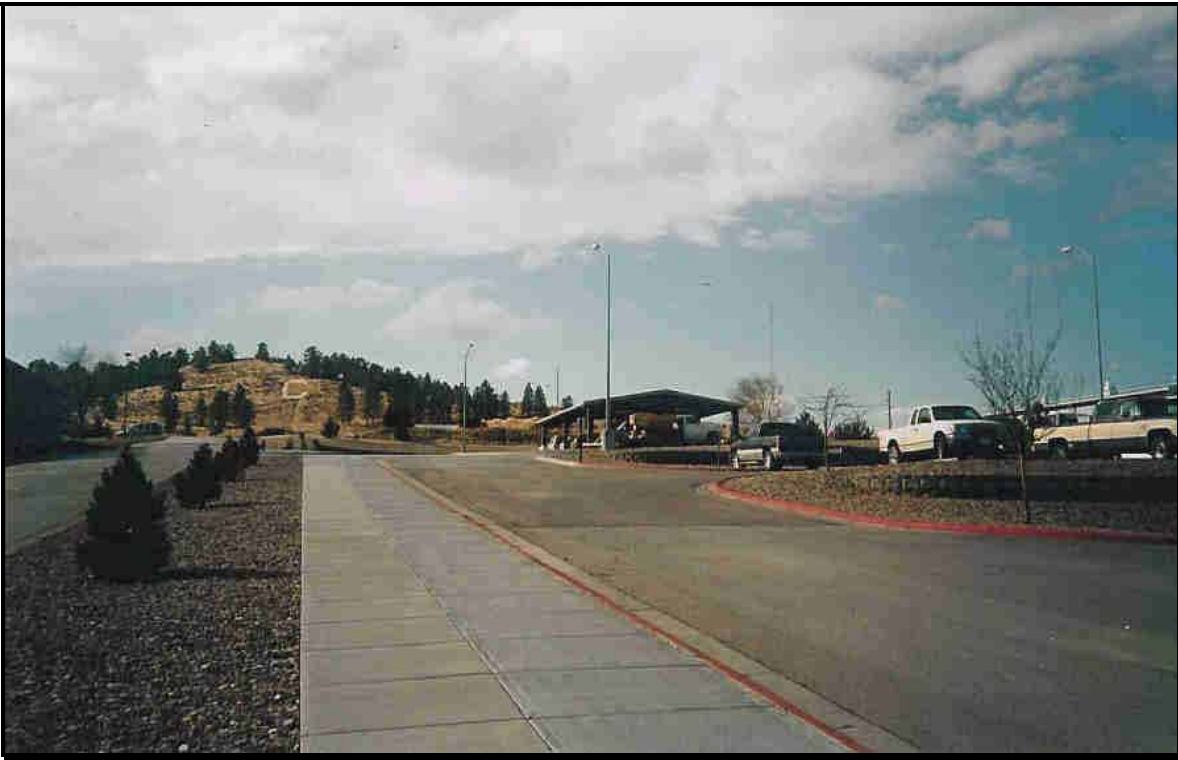
Photo 3: From front of the plant, turn 180 degrees and look south. Open ship storage pile shows off left edge of the shed roof. Pile is about 150 yards from heating plant. Plant is fed by front-end loader as needed.
