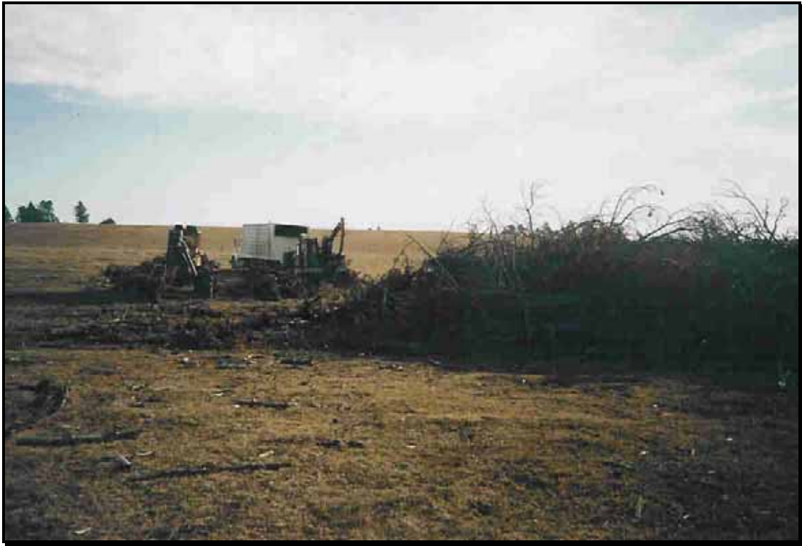
Photo 15: New pile with skidder tearing it apart and feeding the chipper.
