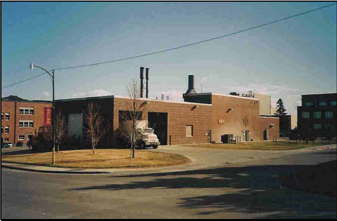
Photo 1: Chadron State College's heating/cooling plant. Fuels storage and biomass boilers are in near portion, original gas boilers in center, and absorption chiller in far end. Cooling tower shows above far end. Front-end loader in shadow at left is used to feed the plant from open storage pile. Bucket holds 1 ton.
